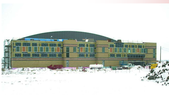
The New Viking Carena under construction.
